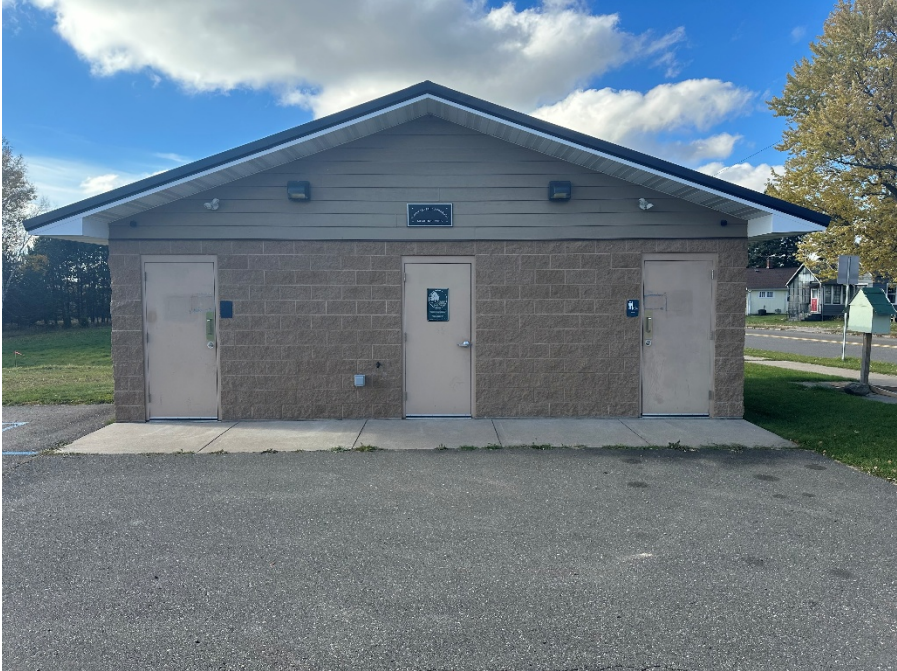
Swede Anderson Recreation Park – Looking west the Restroom Facility.
